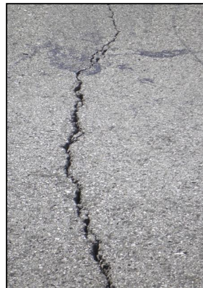
Figure D8.4. Low severity TC (WMA-RAS) Figure D8.5. High severity TC (HMA-RAS)
