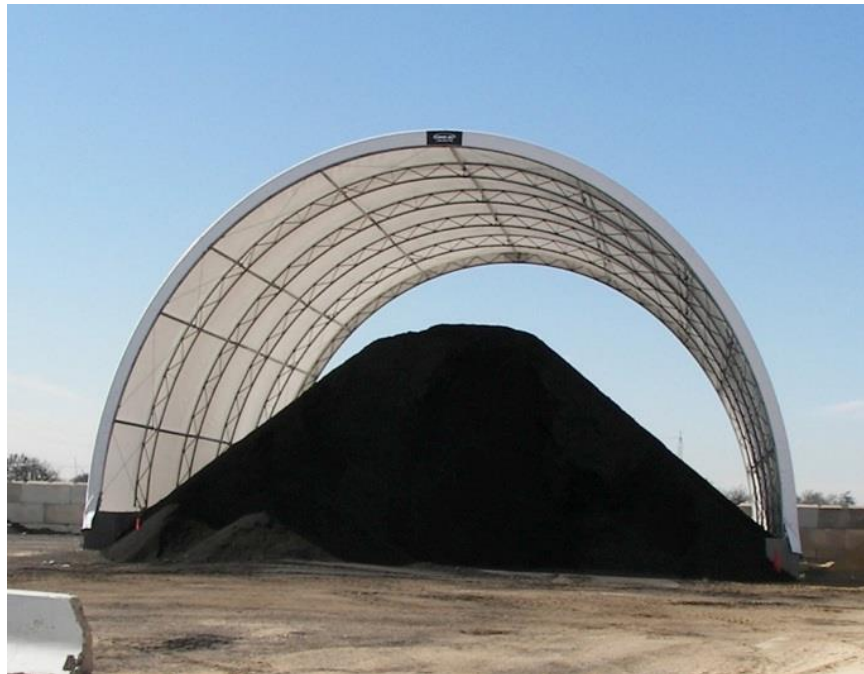
Figure 3. Covered RAS stockpile
