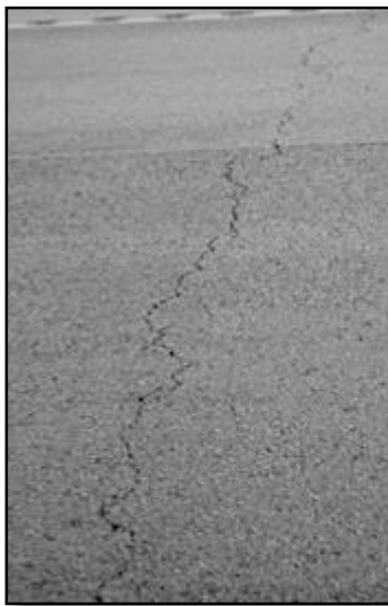
Figure A8.4. Low severity TC (Fine RAS)
