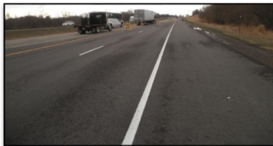
Figure C8.8. Medium raveling west transition
