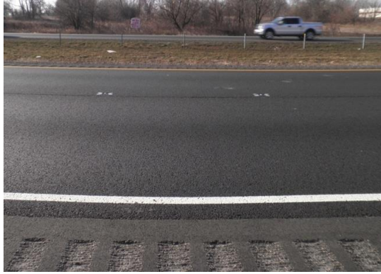
Figure G8.1. EB lane I-80 mile 135.5
