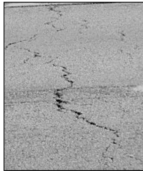
Figure A8.5. Medium severity TC (Control)
