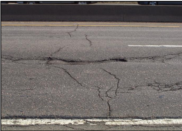
Figure F8.1. Precondition survey (2011) (westbound lane)
