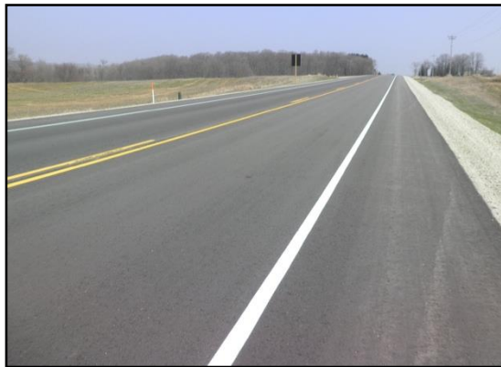
Figure E8.4. Northbound lane HMA with Evotherm® STA 1205+00
