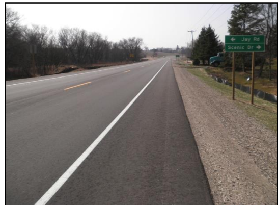
Figure E8.5. Southbound lane HMA with Evotherm® STA 1282+00
