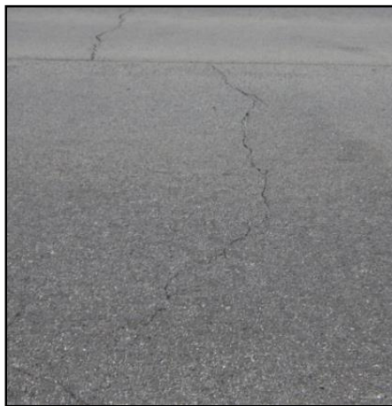
Figure D8.4. Low severity TC (WMA-RAS) Figure D8.5. High severity TC (HMA-RAS)
