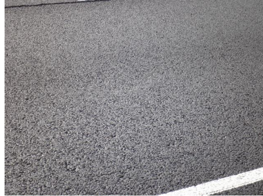
Figure G8.2. WB lane I-80 mile 124.0
