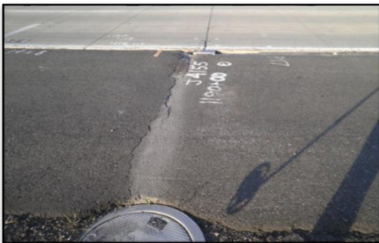
Figure C8.4. Transverse crack Cell 14
