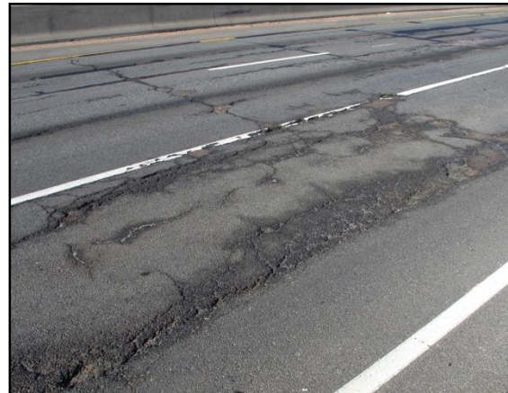
Figure F8.2. Precondition survey (2011) (eastbound lane)
